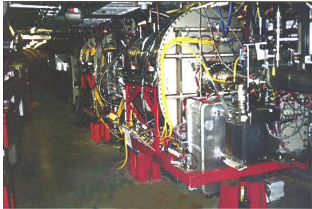
Figure 3. Photo of E1 and E2 cryomodules in the CESR tunnel.
